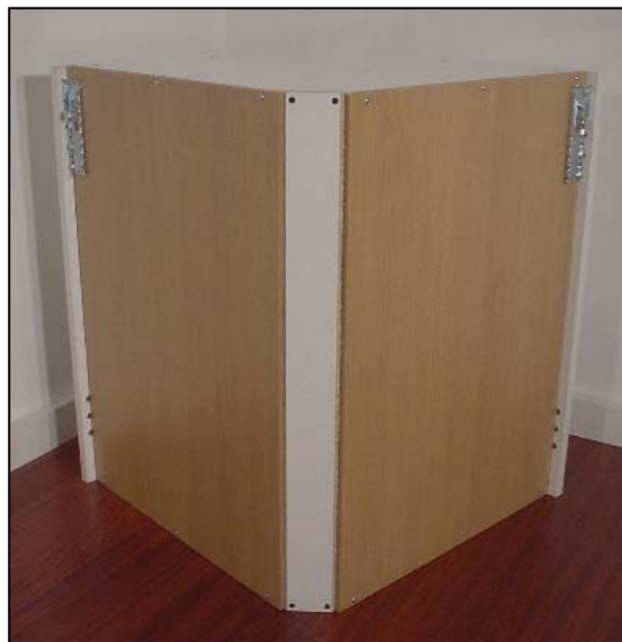
8.3. Secure both hanging brackets
