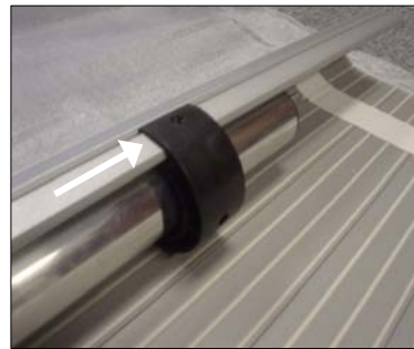
9.1. Slide spring roller onto carpet
